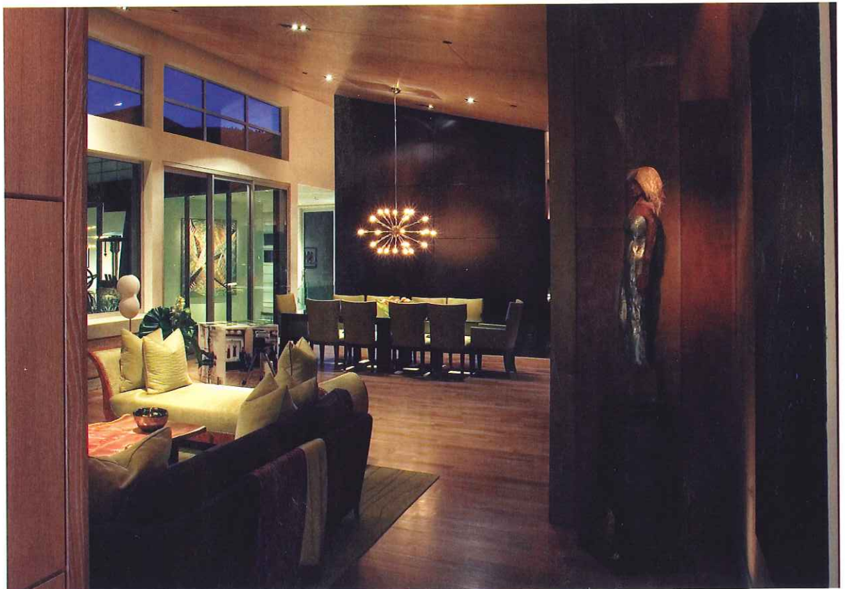
Tiny aperture recessed uplighting highlights the open floor plan from the living room into the dining room. By creating a linear reveal and floating the ceiling, the rammed earth appears as if it extends infinitely. Using a tight beamspread, a recessed wall sculpture is highlighted from above with multi-lamp RSA Combolight CO series recessed square aperture downlighting. Ambient illumination is created by decorative elements as well as multi-lamp RSA Combolight CO series square aperture downlights.
